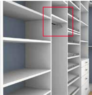
**STEP 1.** Remove closet rod by lifting from under the rod on one side. Remove rod cups. Use flat head screw driver or putty knife to pry behind the cup if needed.
